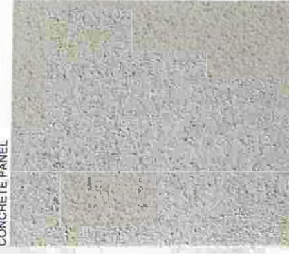
PAINTED/TEXTURED CONCRETE PANEL
