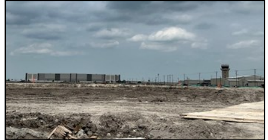
Phase 2 Under Construction
