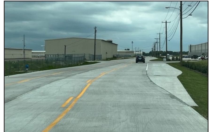
Airport Boulevard Reconstructed
