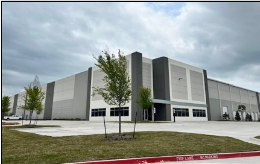
Phase 1 - Building 1 Completed
