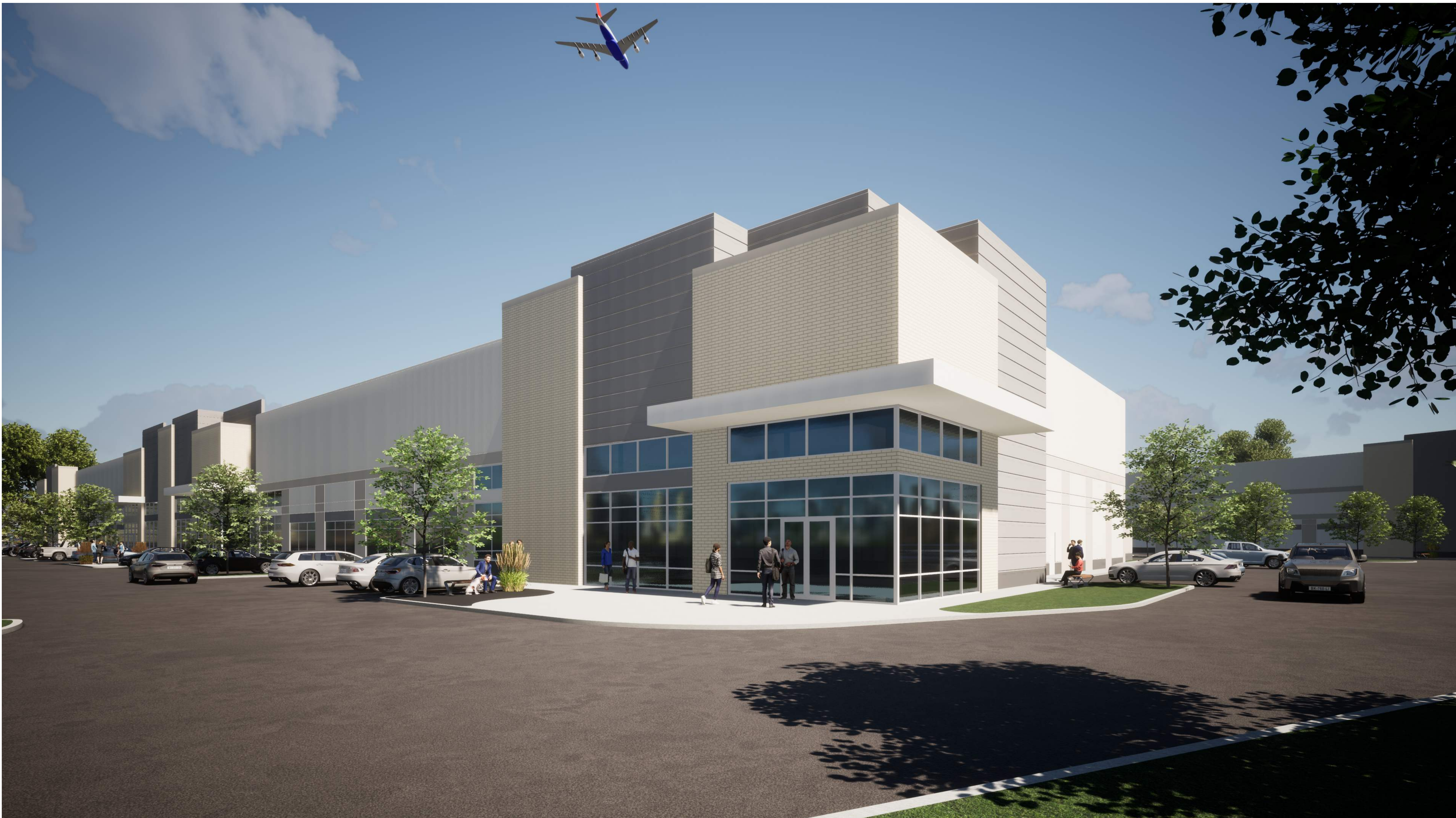
BUILDING "A" NORTHWEST CORNER
