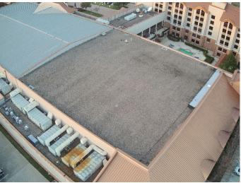
The overall roof of the Mesquite Convention Center appears to be in poor condition. In our professional and unbiased opinion, the roof is retaining abnormal amounts of moisture. This puts the metal structure under the roof in danger of sustaining damage through rust and rot.
