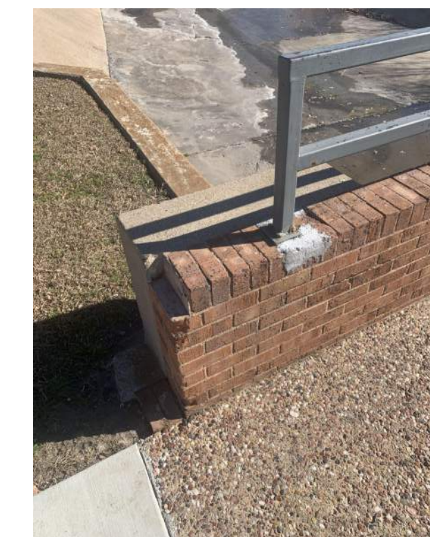
EXISTING BRIDGE CONSTRUCTION
