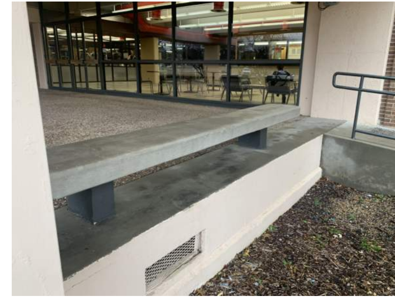
EXISTING ENTRANCE CONSTRUCTION
