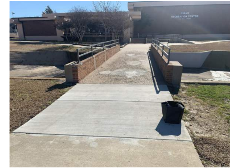
EXISTING BRIDGE CONSTRUCTION
