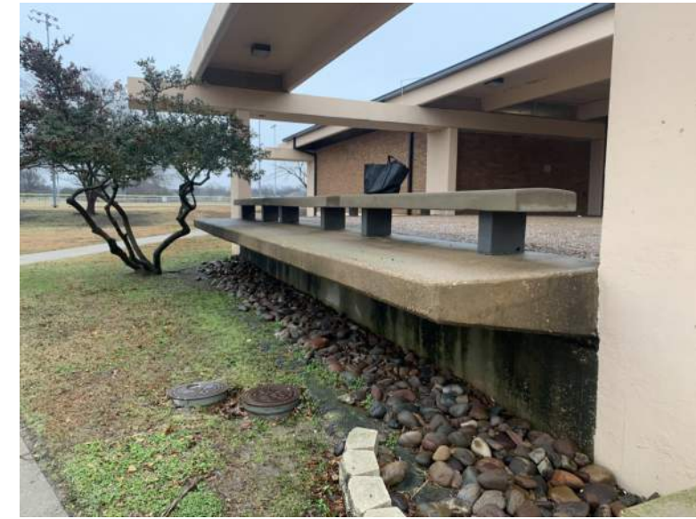
EXISTING ENTRANCE CONSTRUCTION
