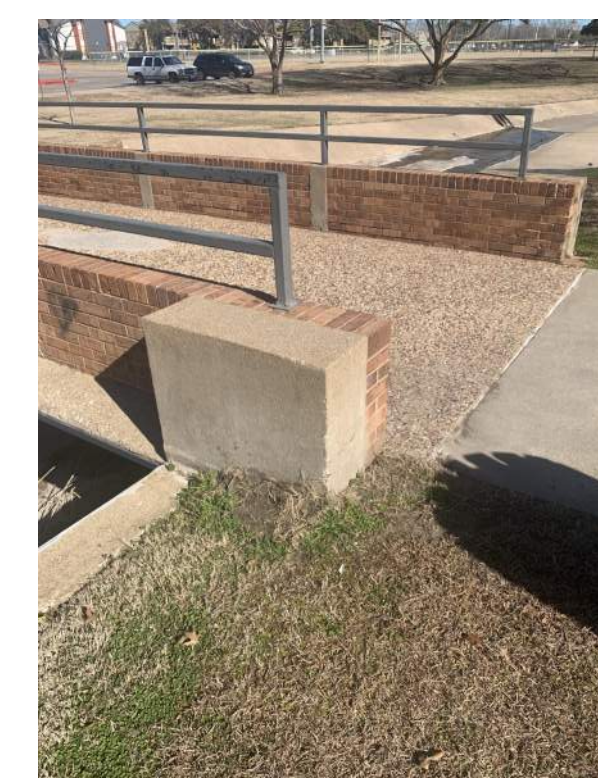
EXISTING BRIDGE CONSTRUCTION
