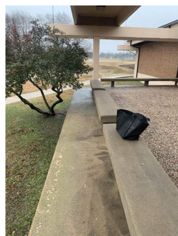
EXISTING ENTRANCE CONSTRUCTION
