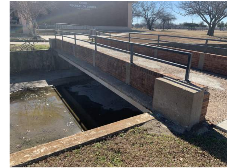
EXISTING BRIDGE CONSTRUCTION
