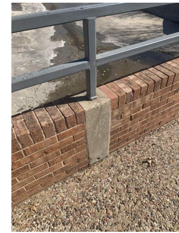
EXISTING BRIDGE CONSTRUCTION
