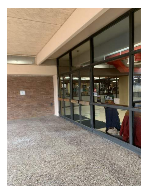
EXISTING ENTRANCE CONSTRUCTION
