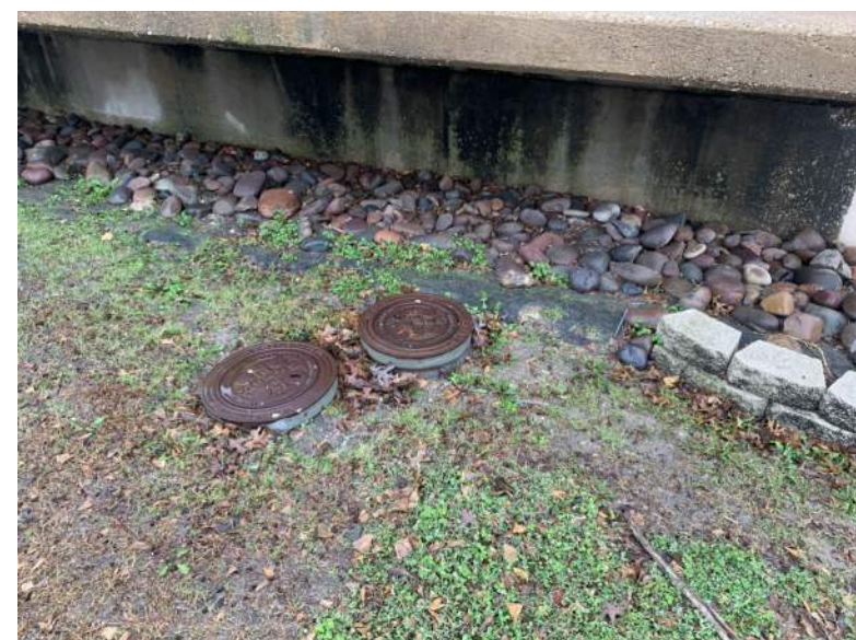
EXISTING ENTRANCE CONSTRUCTION
