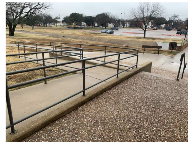
EXISTING ENTRANCE CONSTRUCTION
