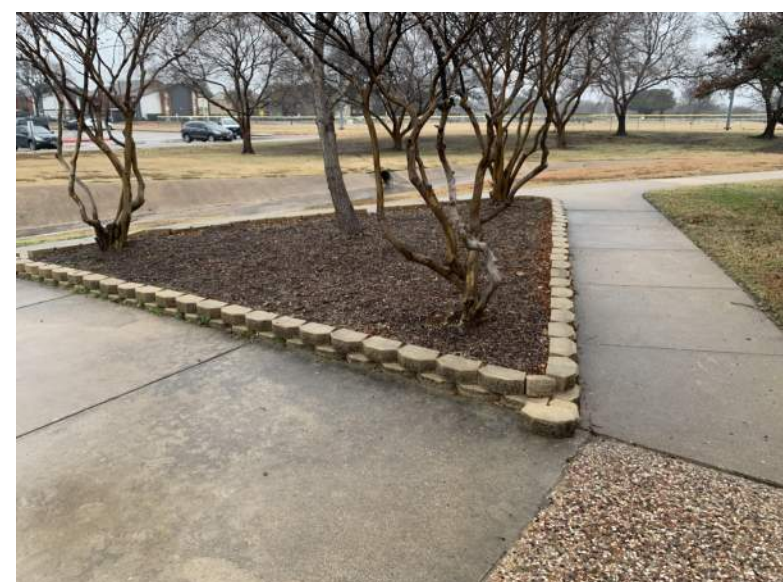
EXISTING ENTRANCE CONSTRUCTION
