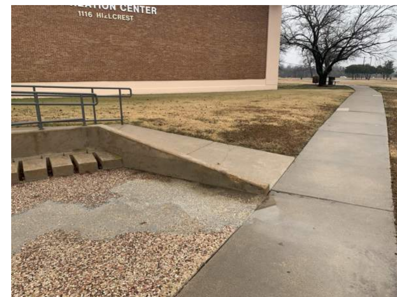
EXISTING ENTRANCE CONSTRUCTION
