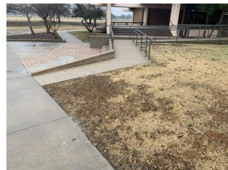
EXISTING ENTRANCE CONSTRUCTION
