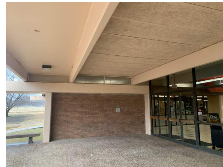
EXISTING ENTRANCE CONSTRUCTION
