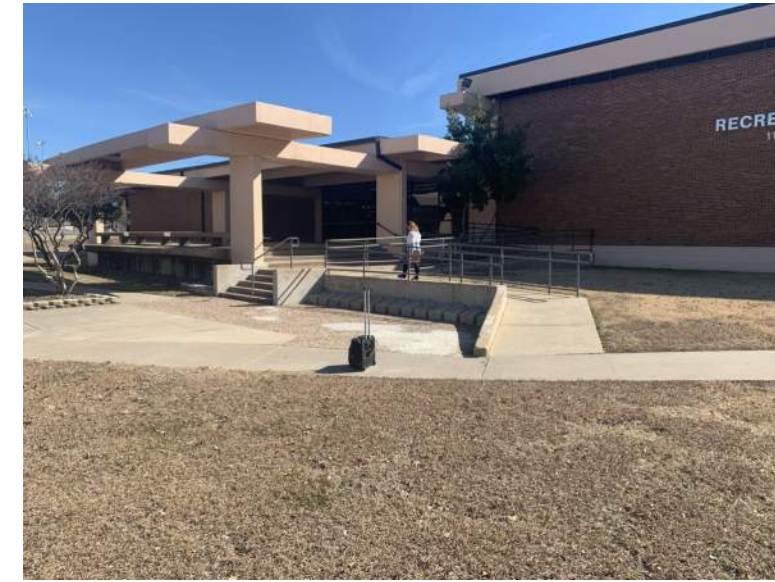
EXISTING ENTRANCE CONSTRUCTION
