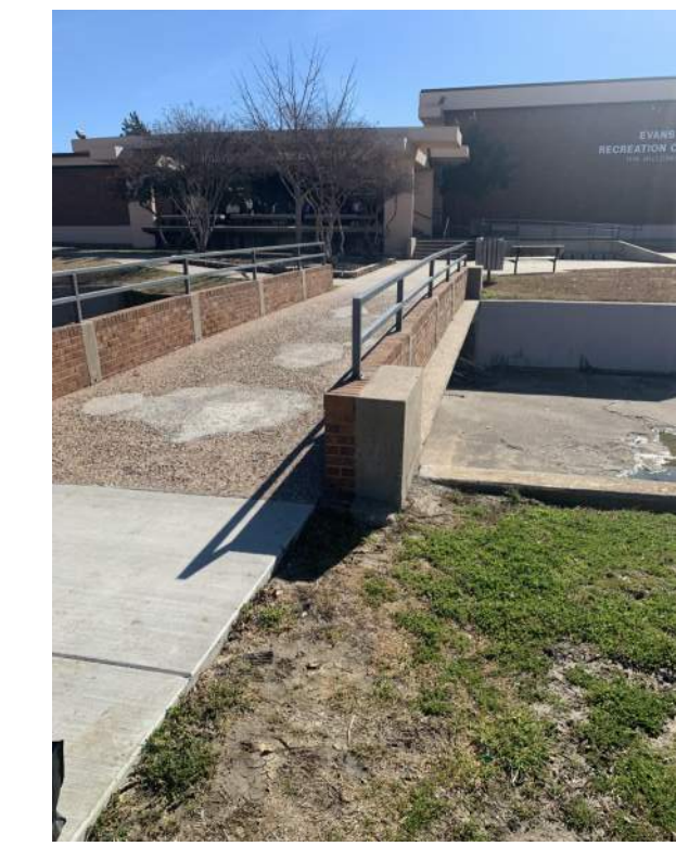
EXISTING BRIDGE CONSTRUCTION
