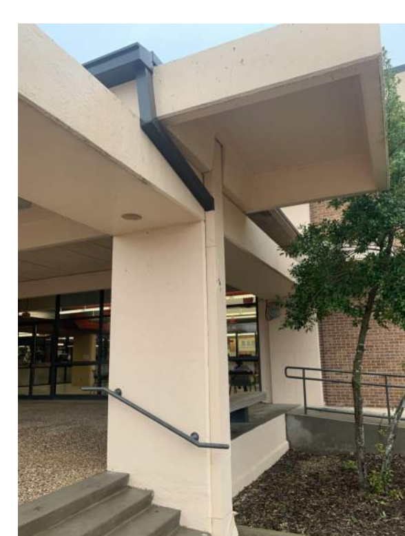
EXISTING ENTRANCE CONSTRUCTION
