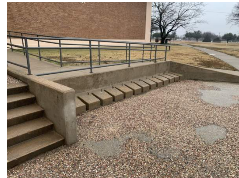
EXISTING ENTRANCE CONSTRUCTION
