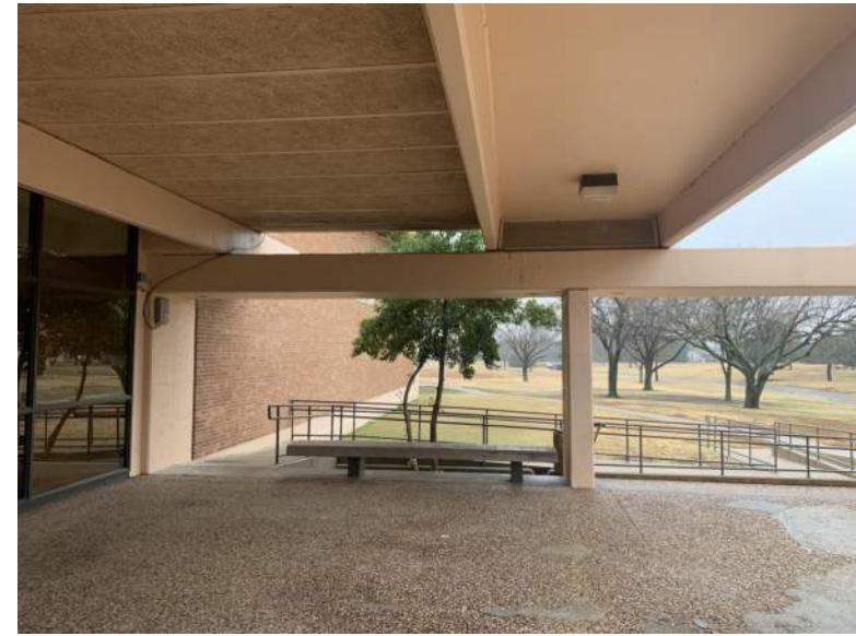
EXISTING ENTRANCE CONSTRUCTION
