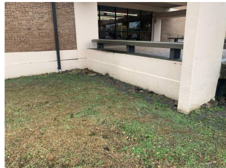
EXISTING ENTRANCE CONSTRUCTION
