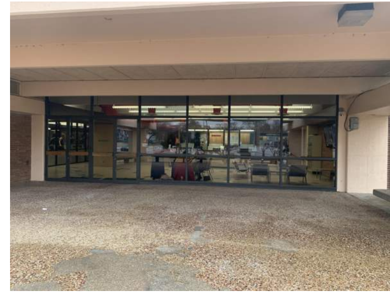
EXISTING ENTRANCE CONSTRUCTION
