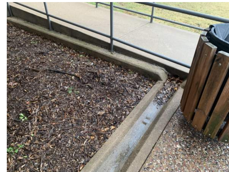
EXISTING ENTRANCE CONSTRUCTION
