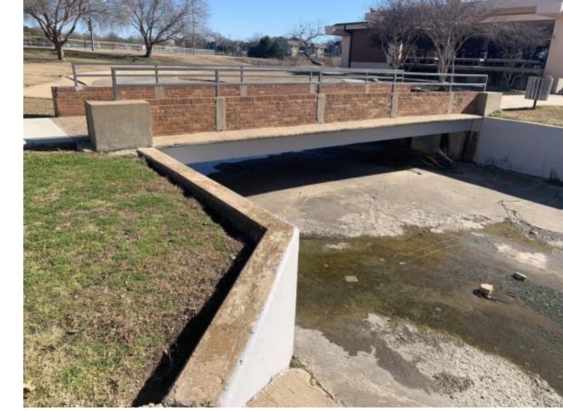
EXISTING BRIDGE CONSTRUCTION
