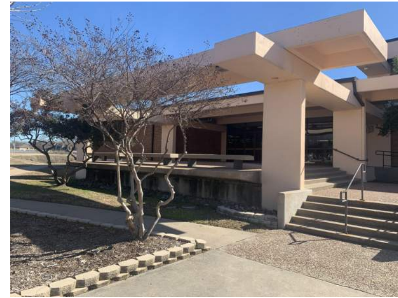
EXISTING ENTRANCE CONSTRUCTION
