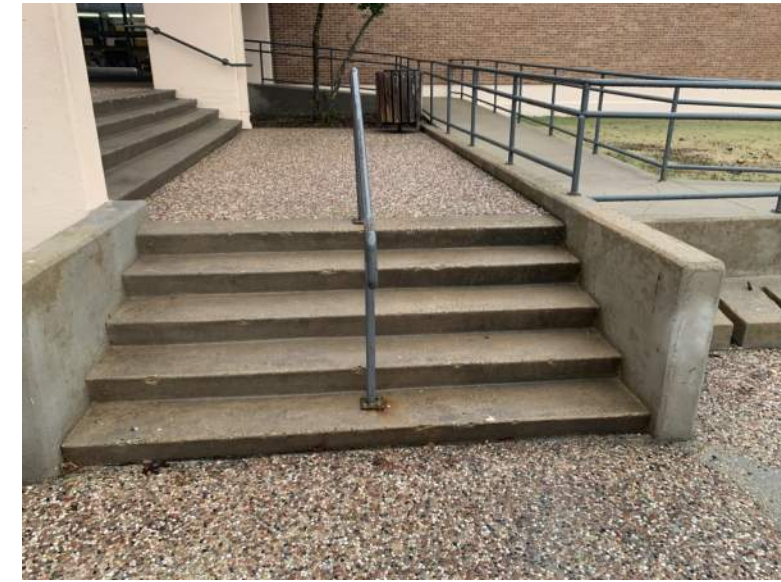
EXISTING ENTRANCE CONSTRUCTION
