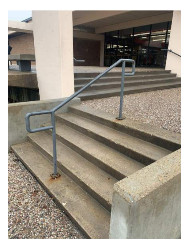
EXISTING ENTRANCE CONSTRUCTION
