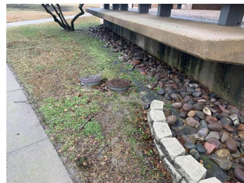
EXISTING ENTRANCE CONSTRUCTION
