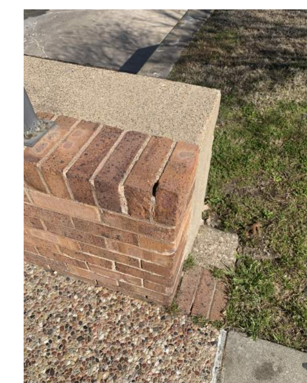
EXISTING BRIDGE CONSTRUCTION
