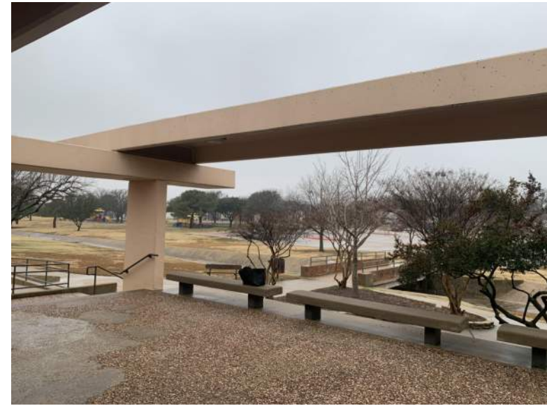
EXISTING ENTRANCE CONSTRUCTION
