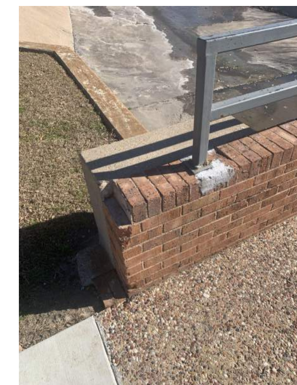
EXISTING BRIDGE CONSTRUCTION
