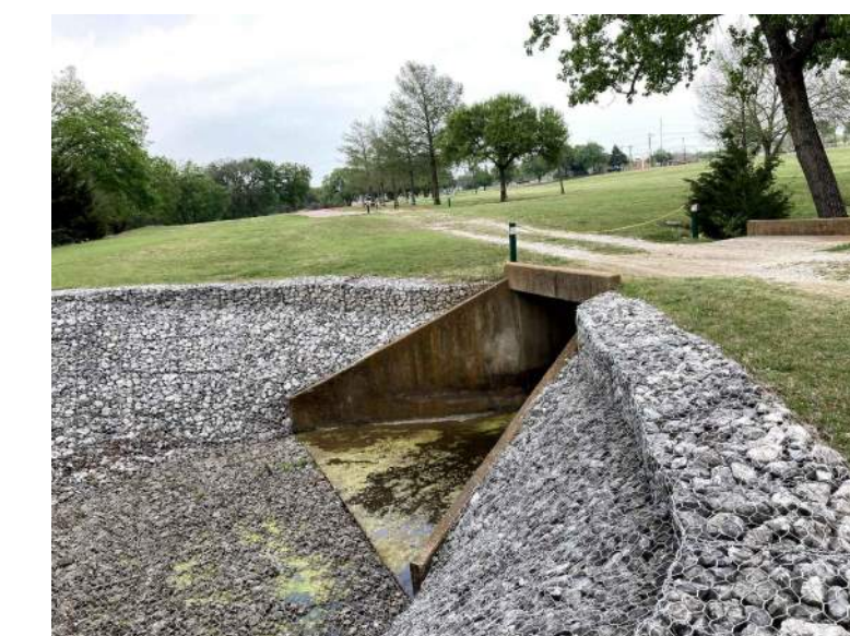
ACCESS FOR JUNCTION BOX AT SM 6183 BRIDGE CROSSING PHOTO 4
