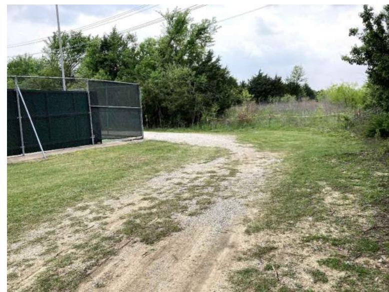
ACCESS FOR JUNCTION BOX AT SM 6183 PHOTO 3
