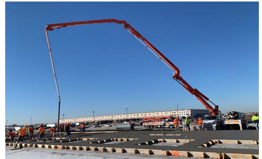
Building 1 Tilt Walls Being Poured
