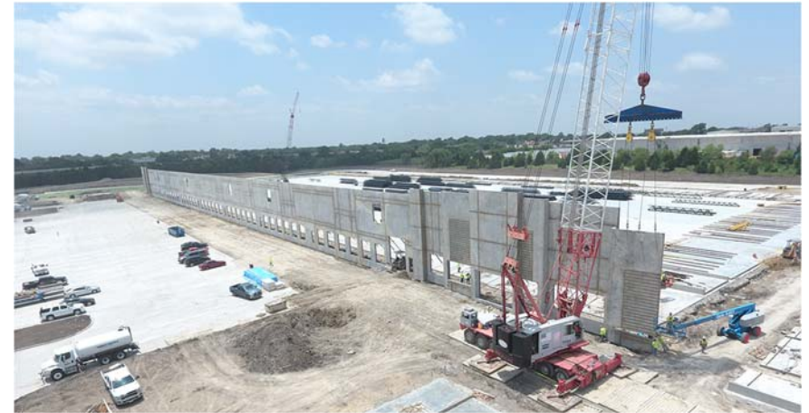
Southwest View of Building 1 Under Construction
