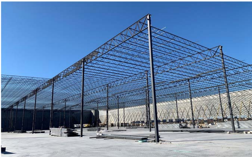
Building 1 Framing Under Construction
