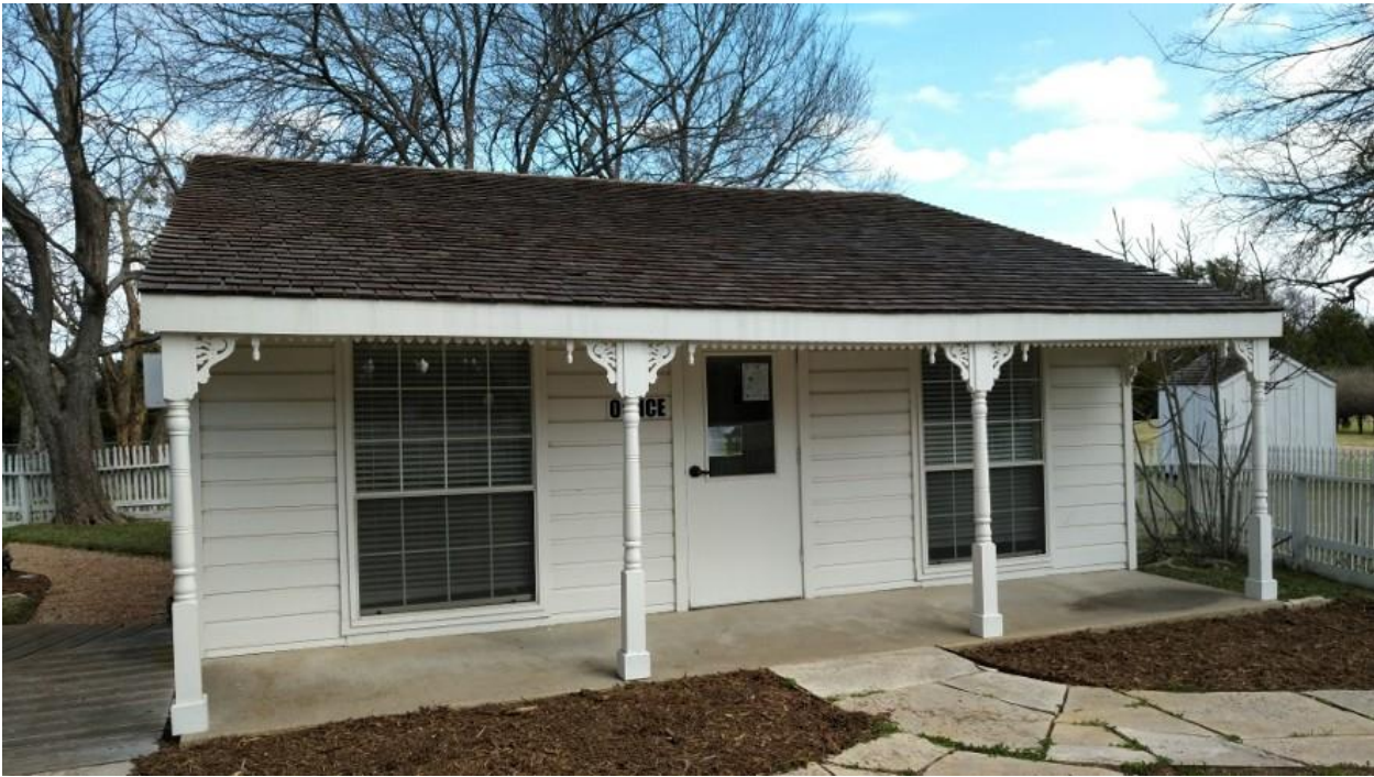
Figure 15. West side of the Florence Ranch Office, 2018
