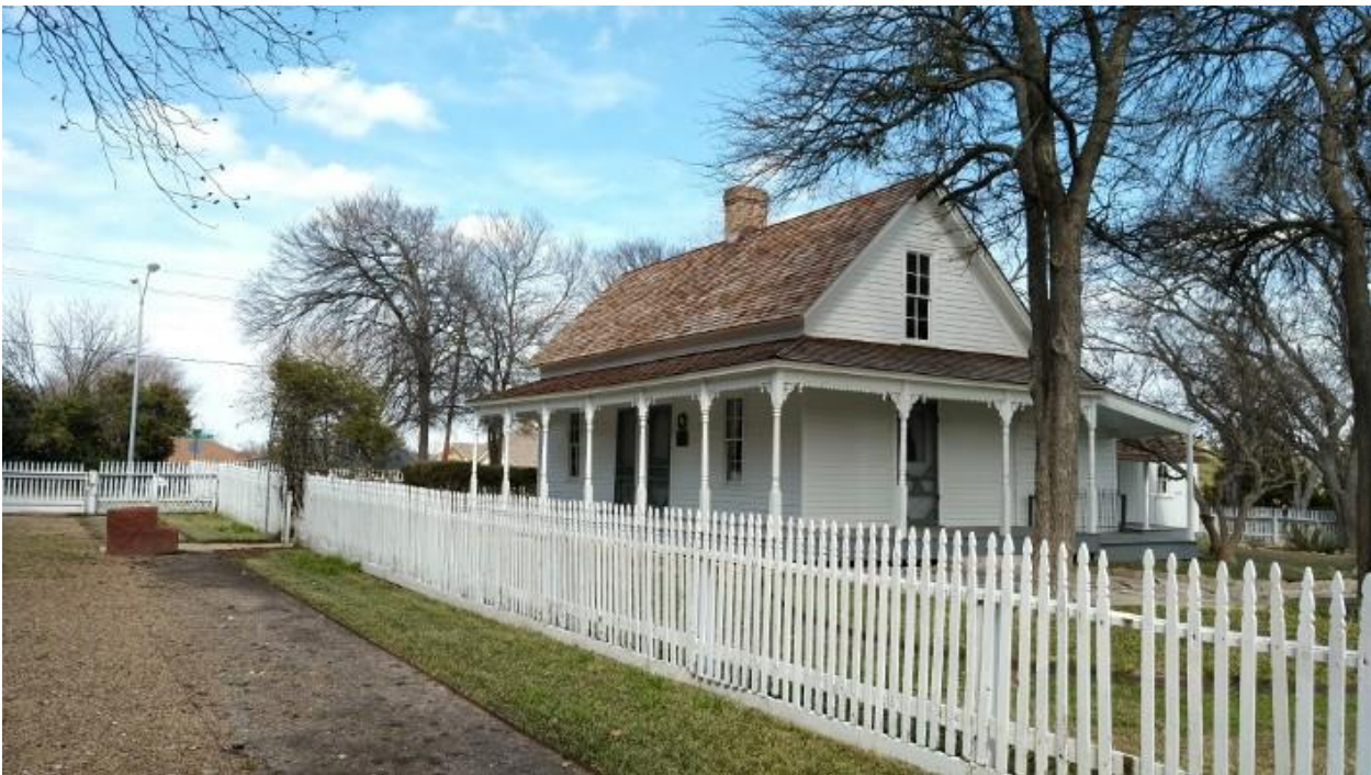
Figure 8. West and south side of Main House, 2018
