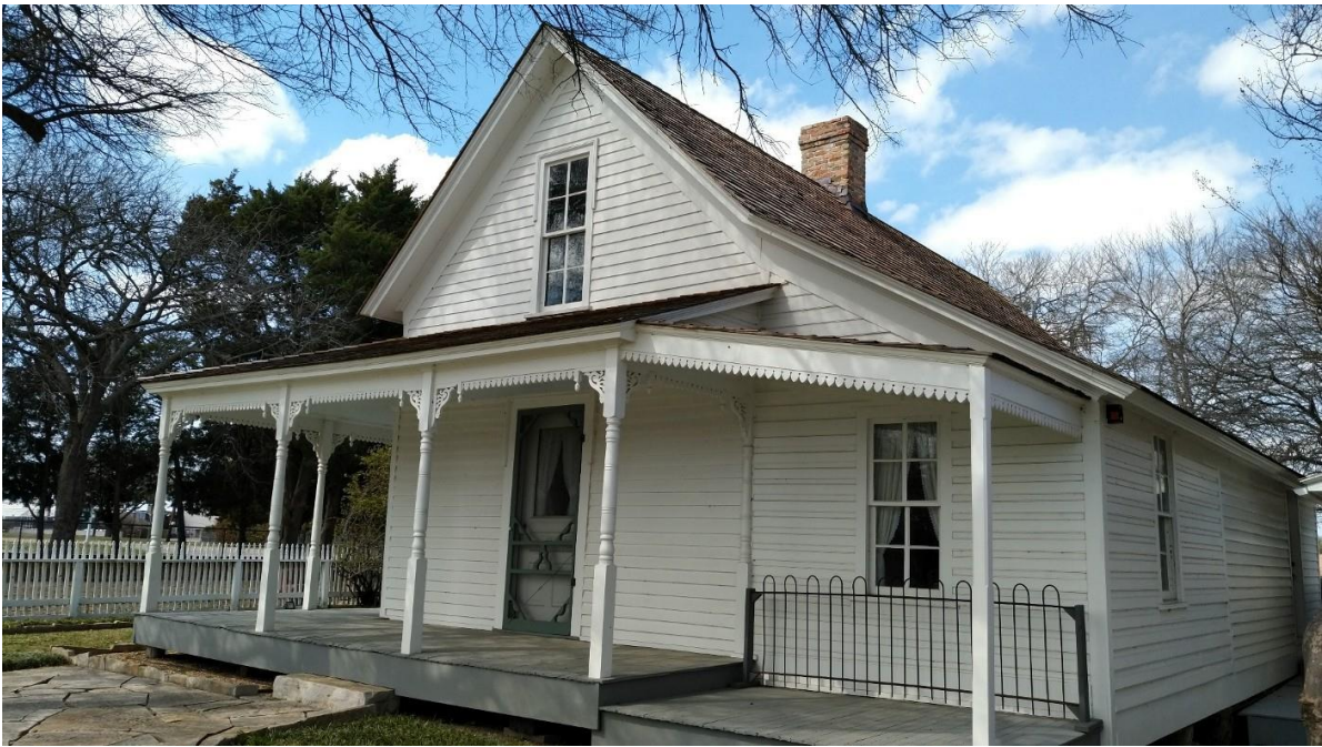
Figure 6. Main House south exterior, 2018
